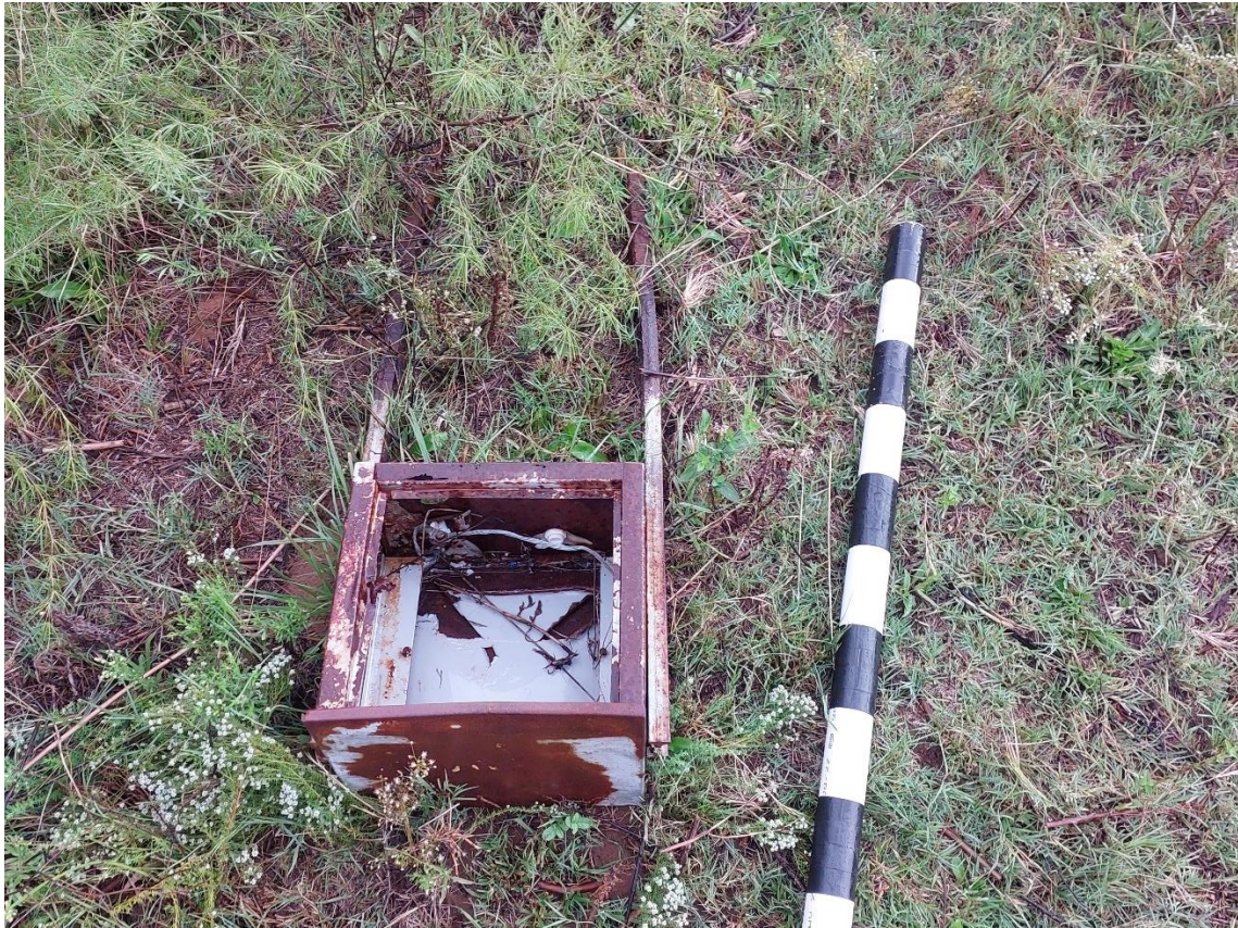
Figure 45: Telephone junction box found at MO002
